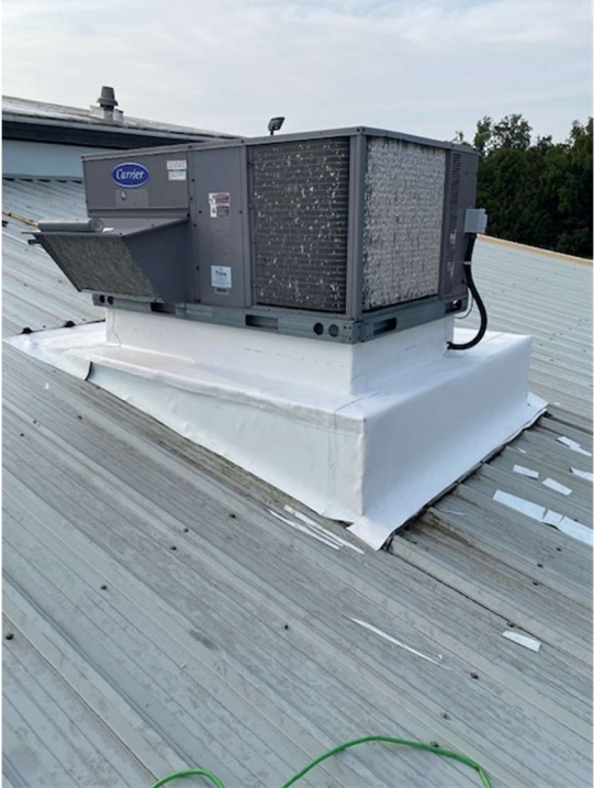
Roof tops wrapped first,
