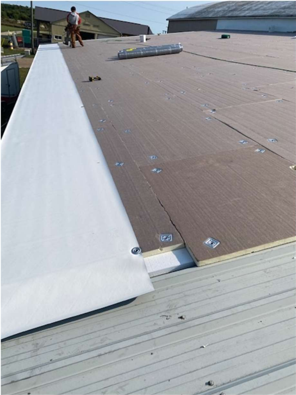
Insulation underlay and first sheet
