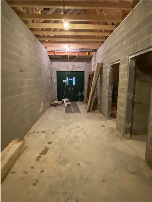
Back hallway to existing hallway
