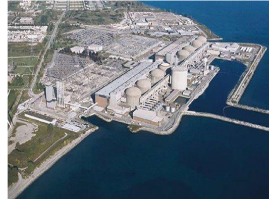
Overview of Pickering Nuclear Generating Station
