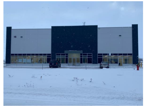
Exterior of the Western Clean Energy Sorting and Recycling Facility
