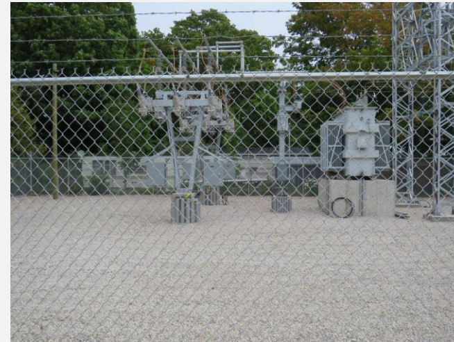
Teeswater Under Construction 2024
