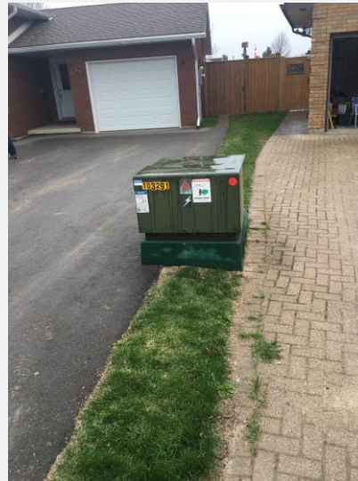
Kincardine Underground Rebuild
