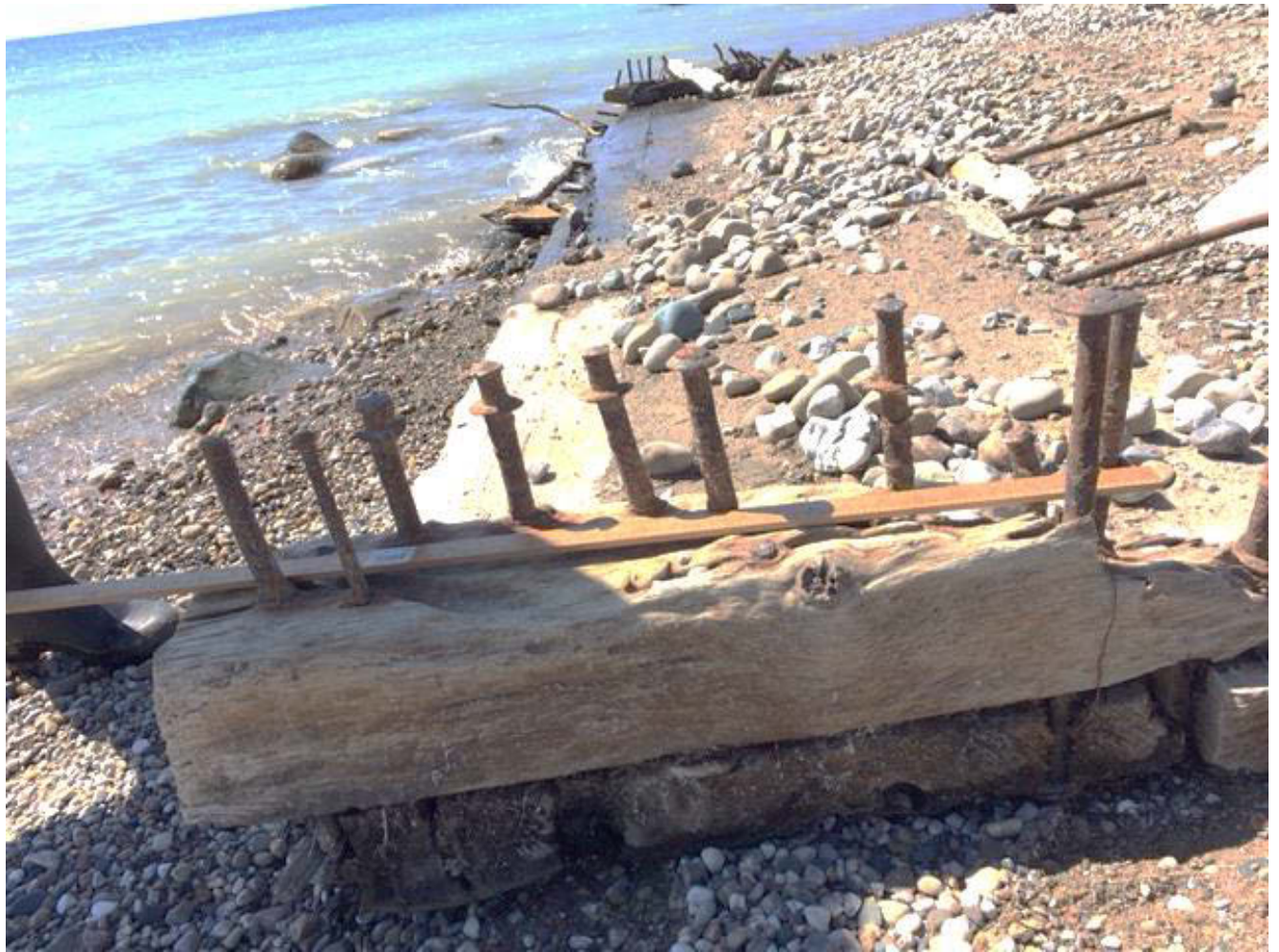
Photograph 8: View of Underlying Planks (May 2021)
