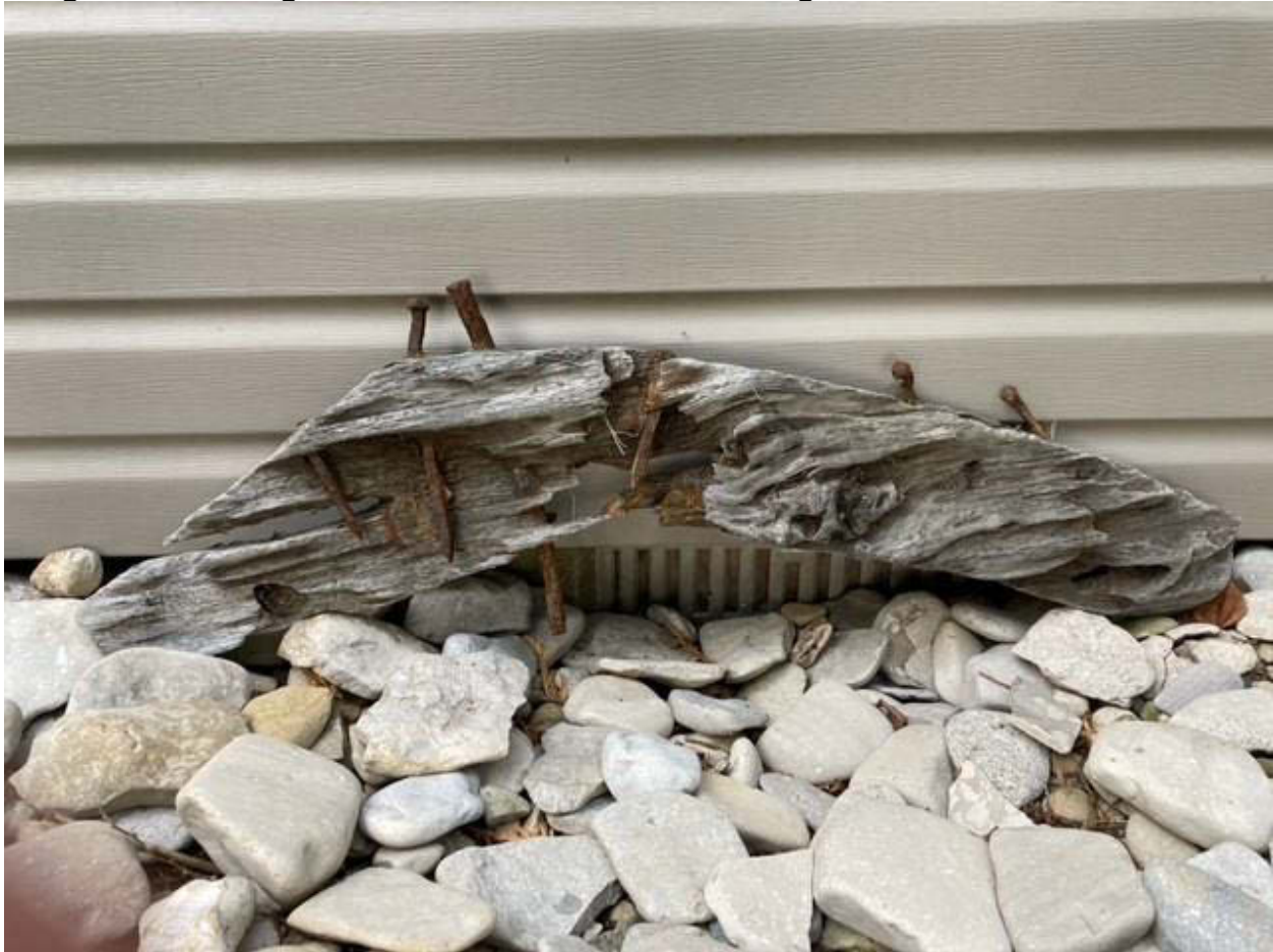
Image 42: Wreckage recovered and located at cottage
