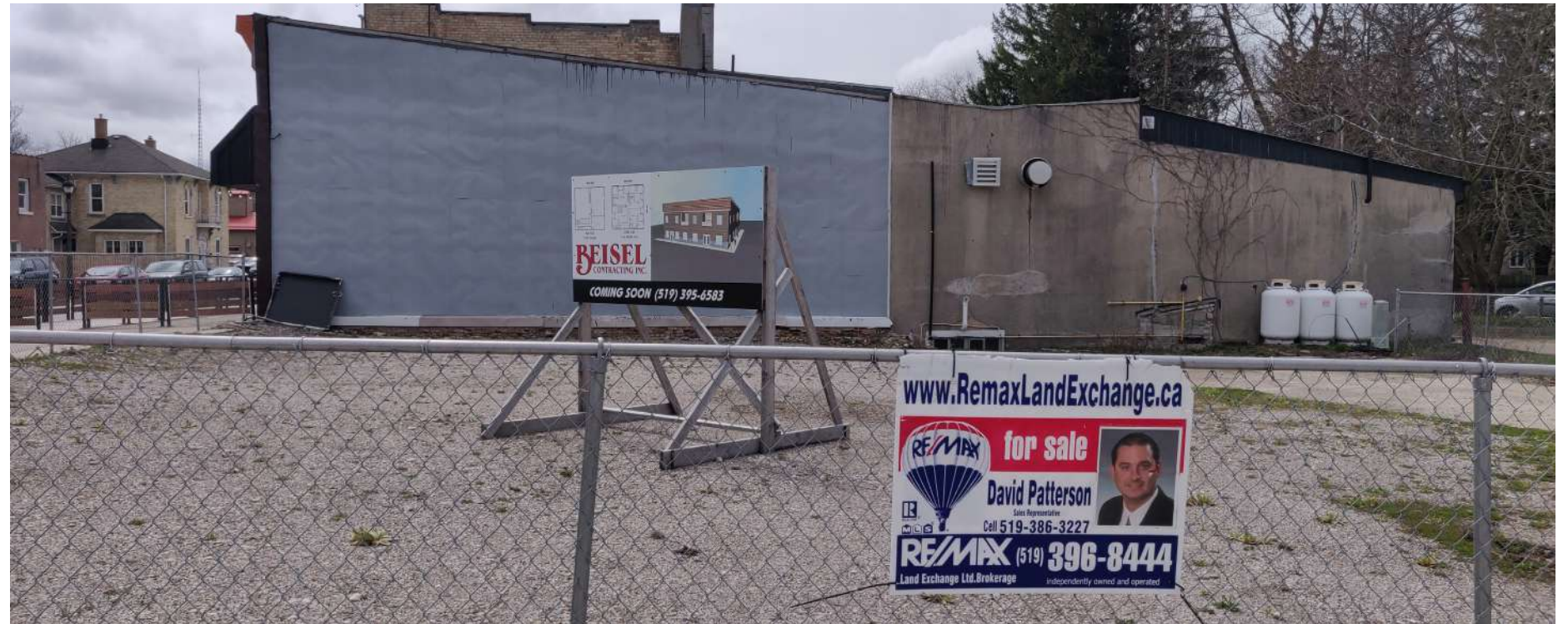
Subject of P1. Vacant Lot, 89 Queen Street Development
