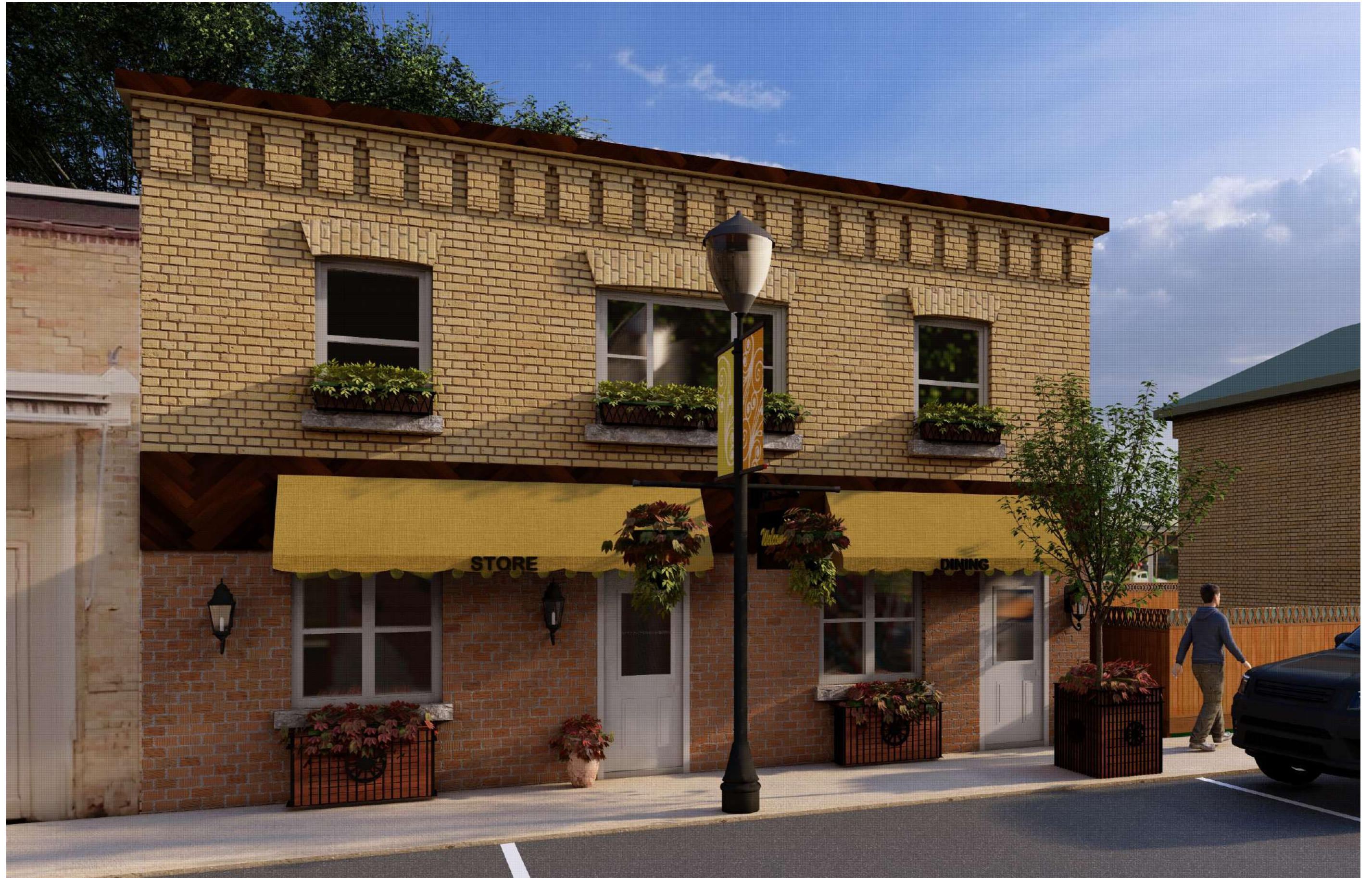
Façade Enhancements at 82 Huron Street
