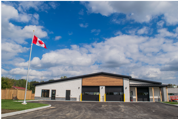
The new paramedic base in September 2025.
