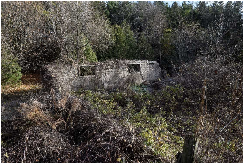
IMAGE 2: AREA OF PREVIOUS DISTURBANCE RELATED TO FORMER BARN, NORTHEAST
